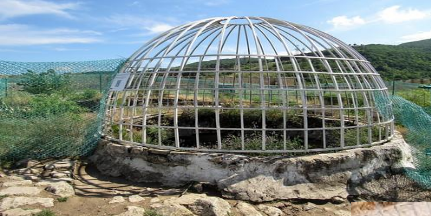
A wire dome installed over a land-covered building
