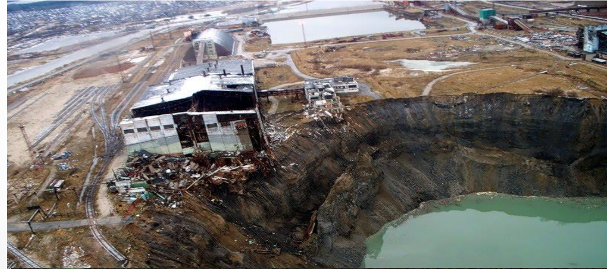
Monitoring of mines
