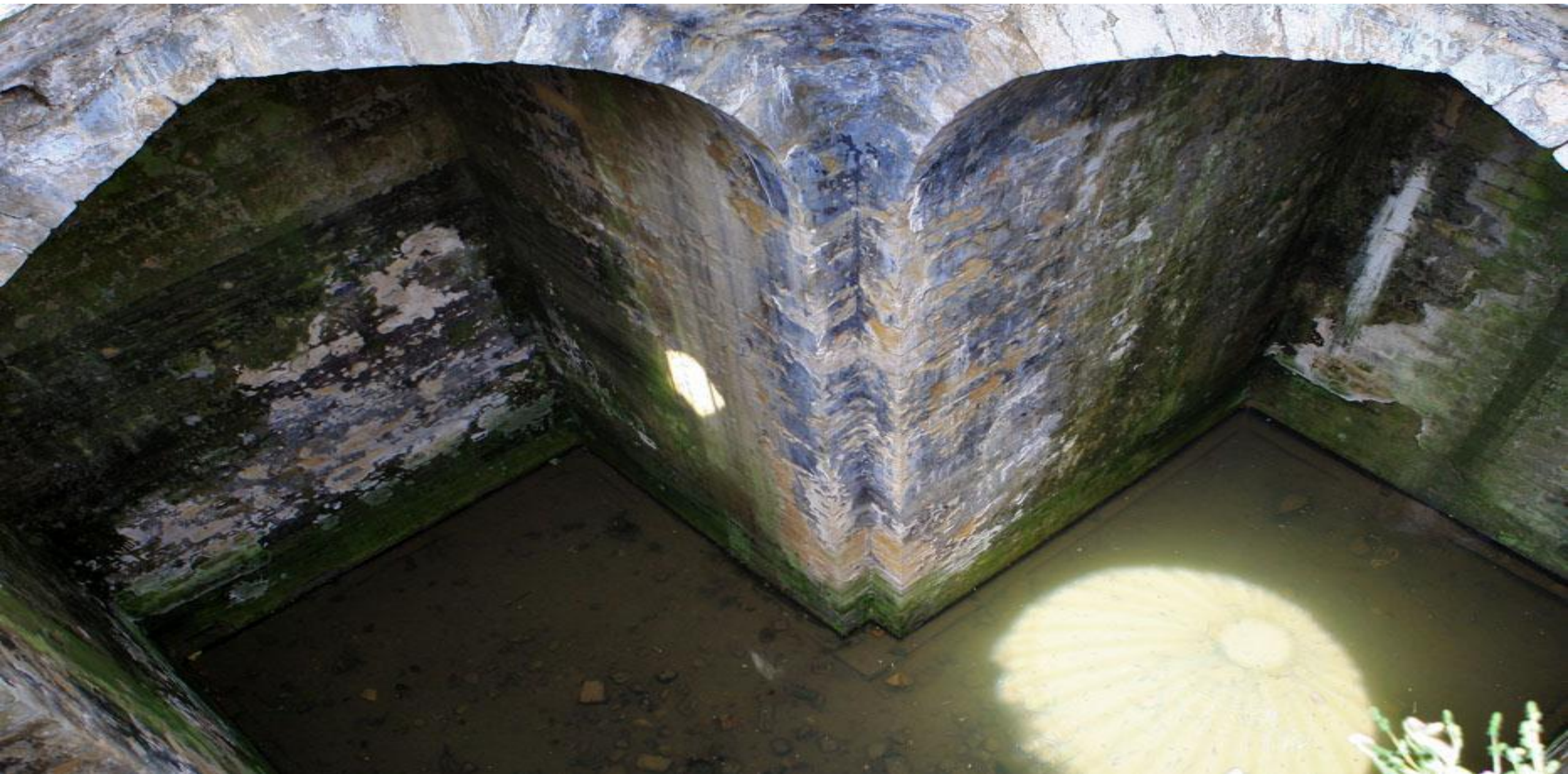
The interior of the building under the wire dome
